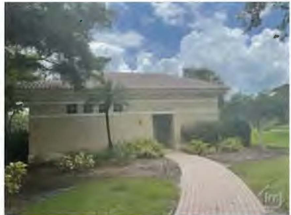
Restroom/Storage Building Taken: 5/24/2022
