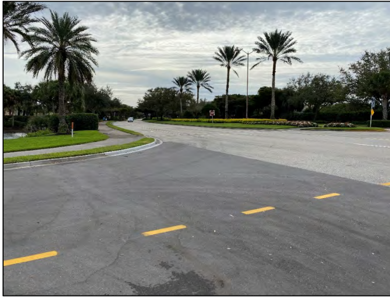
Figure 4-2: Oakwilde Boulevard Southbound Turnout onto Westbound Coconut Road
