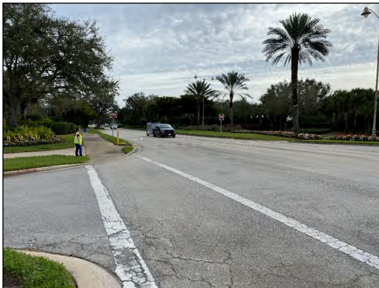
Figure 6-3: The Commons Club Southbound Turnout onto Westbound Coconut Road
