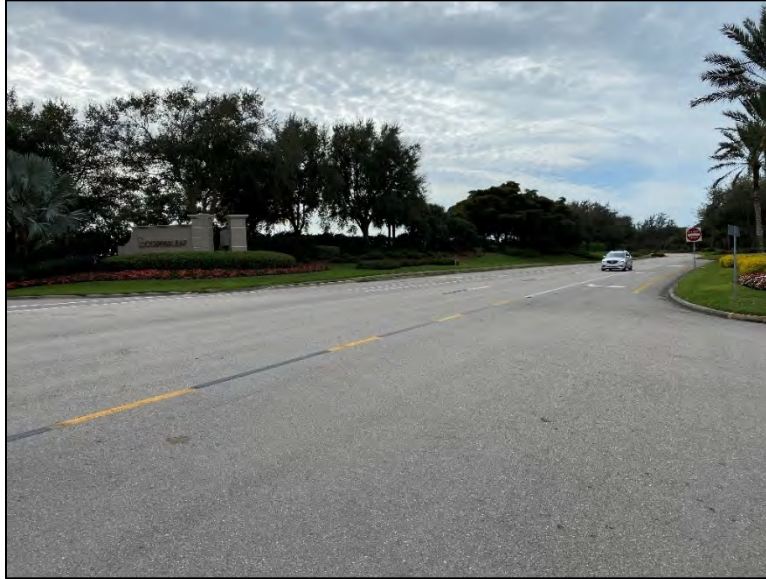
Figure 11-2: Three Oaks Parkway Southbound Left Turn onto Eastbound Copperleaf Boulevard
